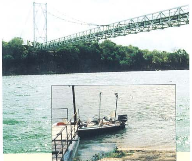
The existing Chirundu Bridge and small boat used for the survey.
