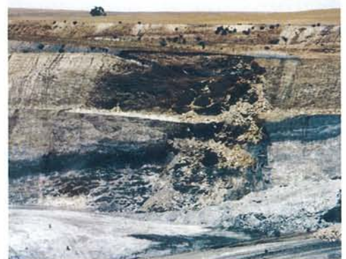
Zoutkloof south-east corner failure in progress.
