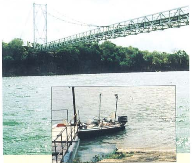
The existing Chirundu Bridge and small boat used for the survey.
