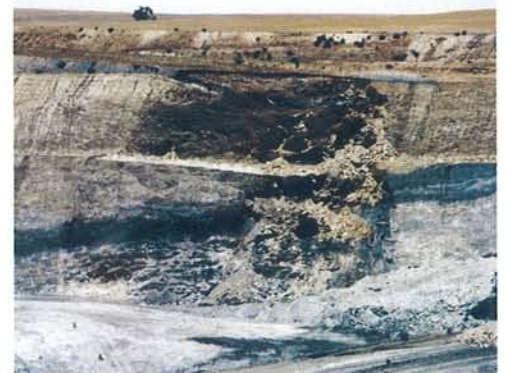
Zoutkloof south-east corner failure in progress.
