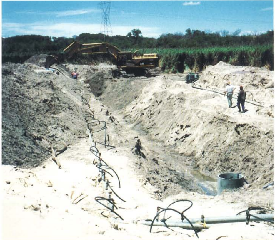
Excavation for a collector well showing dewatering wellpoints.
