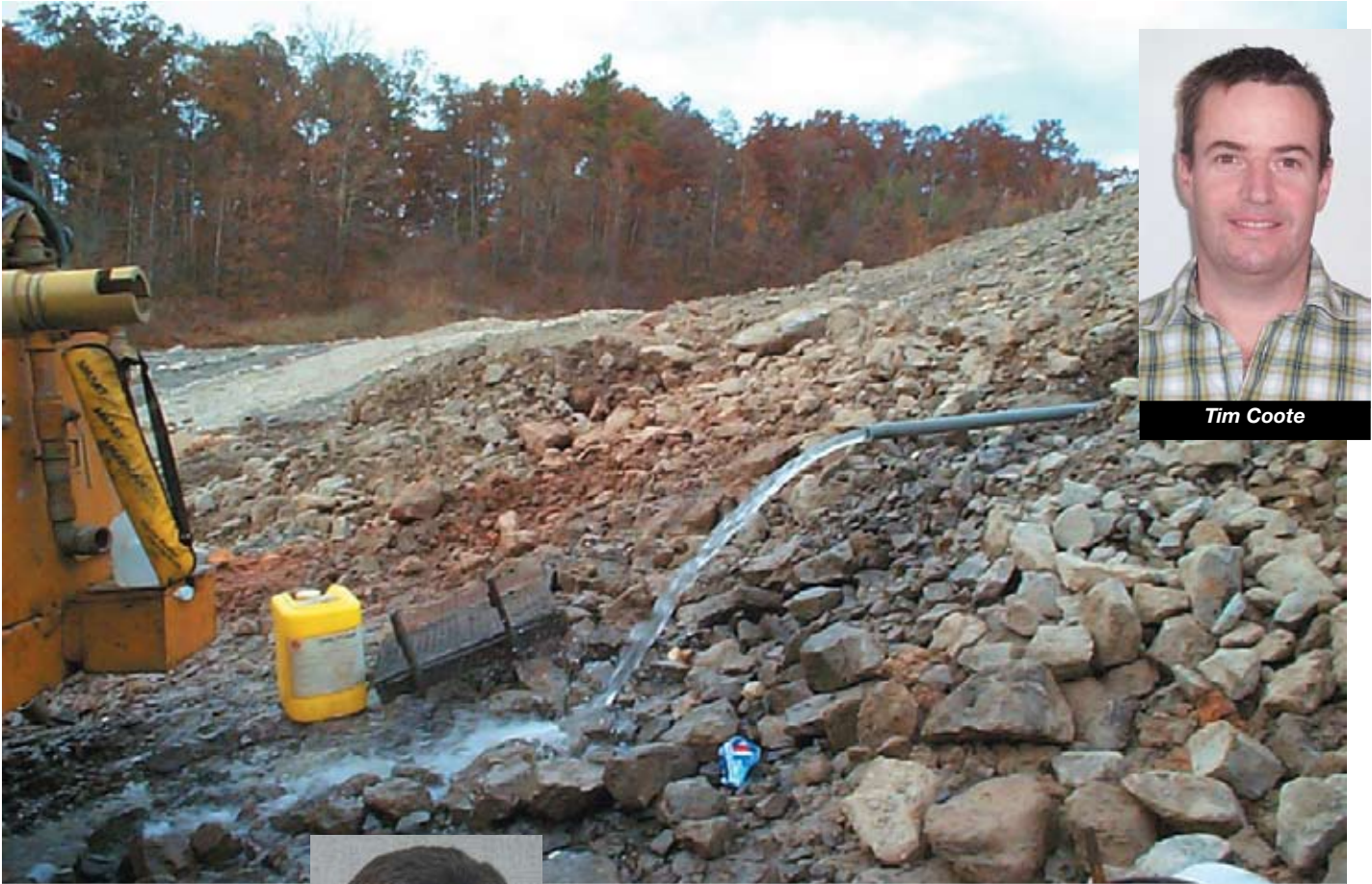
Brushy Creek Tailings Dam - Initial drain flow (DH-1) of 35 GPM
