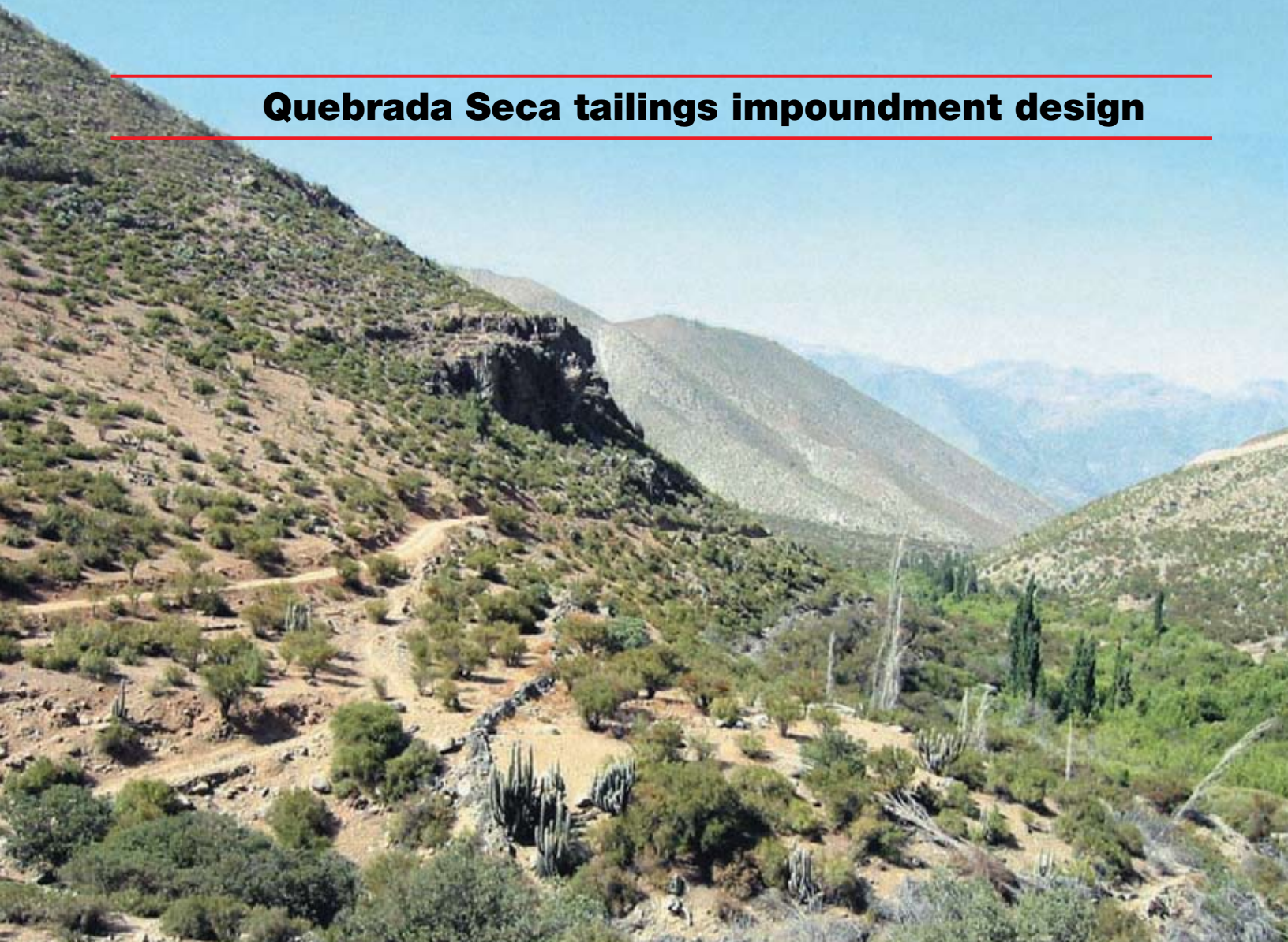
Rio Manque at the Quebrada Seca tailings dam site
