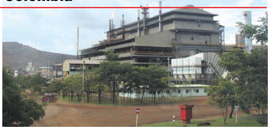
Line 1 and 2 smelters, shortly after expansion. Open pit can be seen in the left background.
