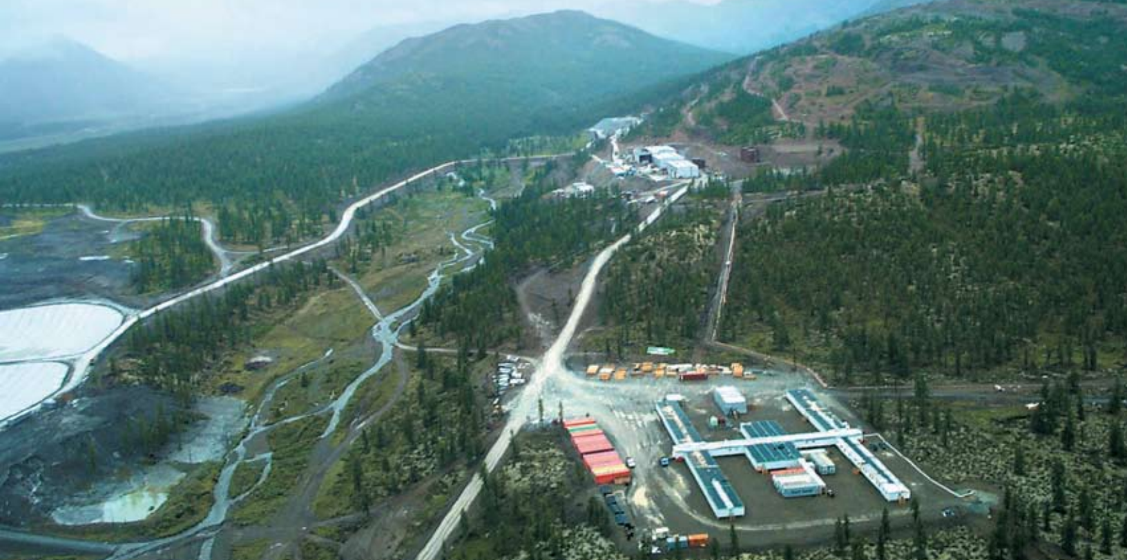
Foreground: man camp, left foreground: tailing impoundments, centre: process plant, background: mine portal
