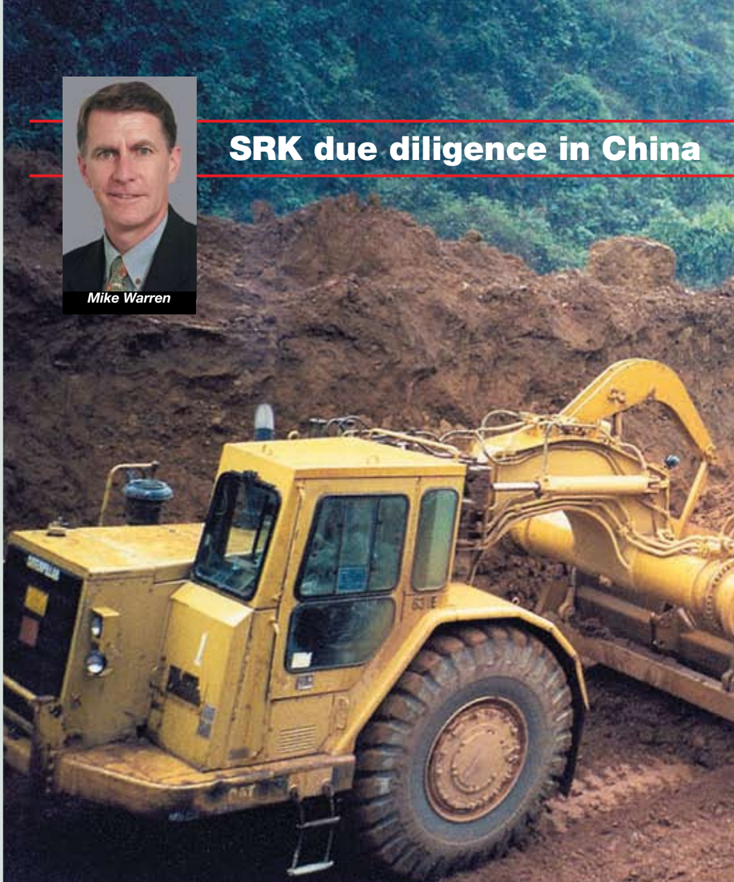
Imported Caterpillar scraper and dozer
