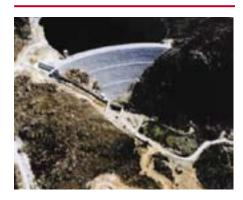
Located on the Koekedouw River upstream of Ceres in the Western Cape, this dam is 62m high and is designed to supply 17 million m<sup>3</sup>/annum (cubics per meter), including a portion allocated to emerging farmers.
