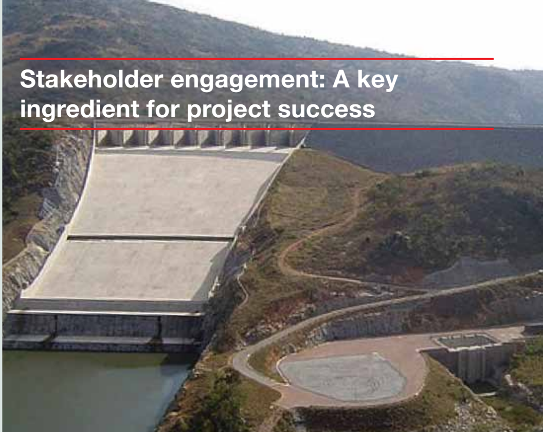
Maguga dam, Swaziland
