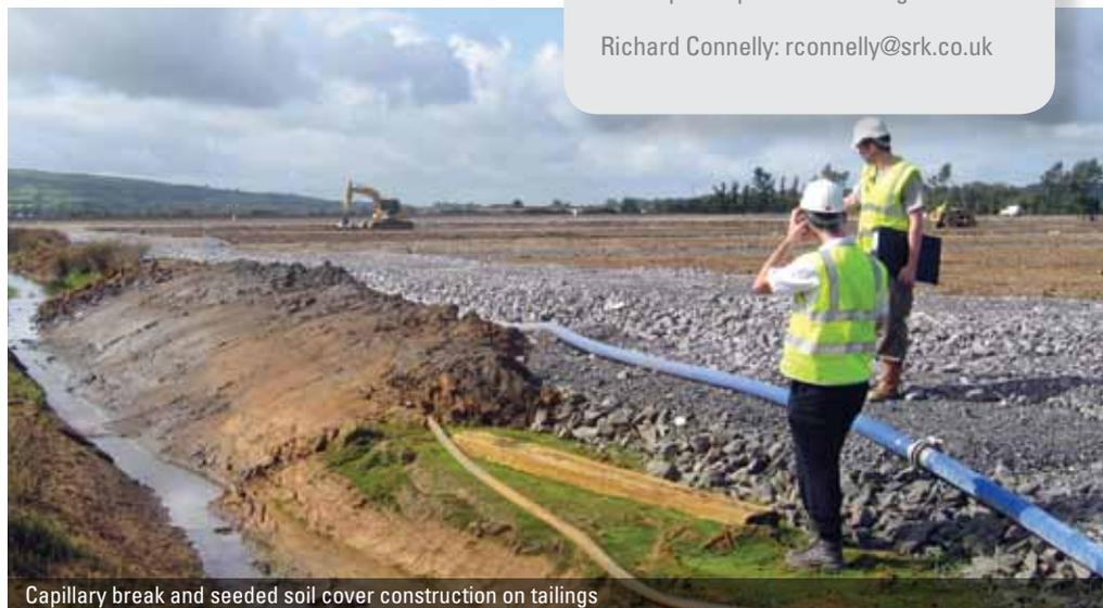
Capillary break and seeded soil cover construction on tailings
