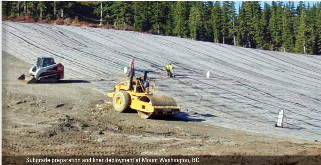
Subgrade preparation and liner deployment at Mount Washington, BC
