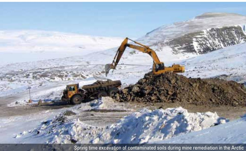
Spring time excavation of contaminated soils during mine remediation in the Arctic
