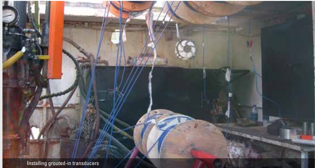
Installing grouted-in transducers
