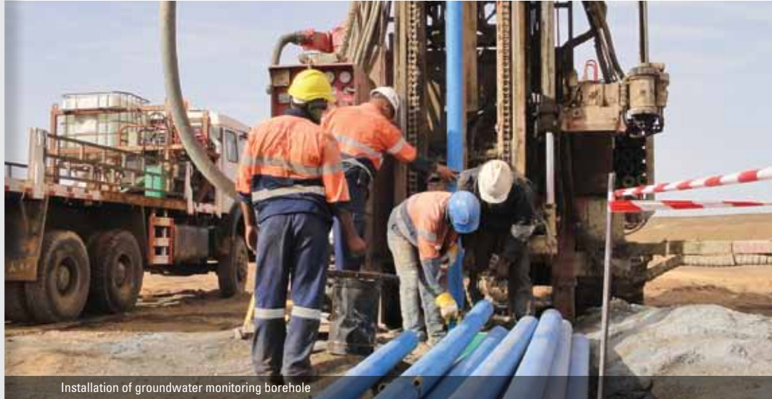
Installation of groundwater monitoring borehole
