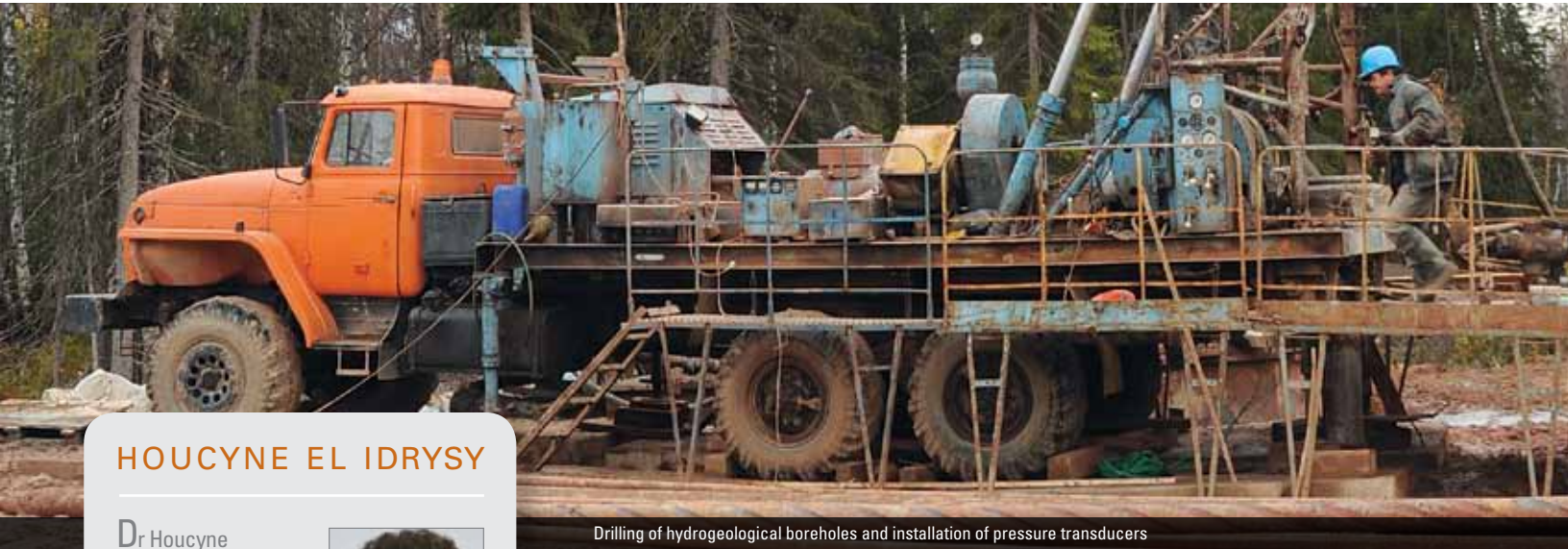
Drilling of hydrogeological boreholes and installation of pressure transducers
