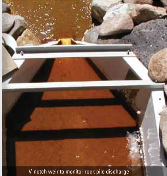
V-notch weir to monitor rock pile discharge
