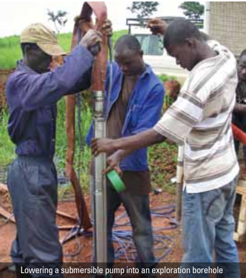
Lowering a submersible pump into an exploration borehole
