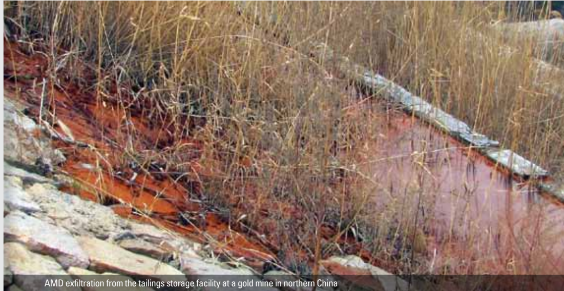
AMD exfiltration from the tailings storage facility at a gold mine in northern China
