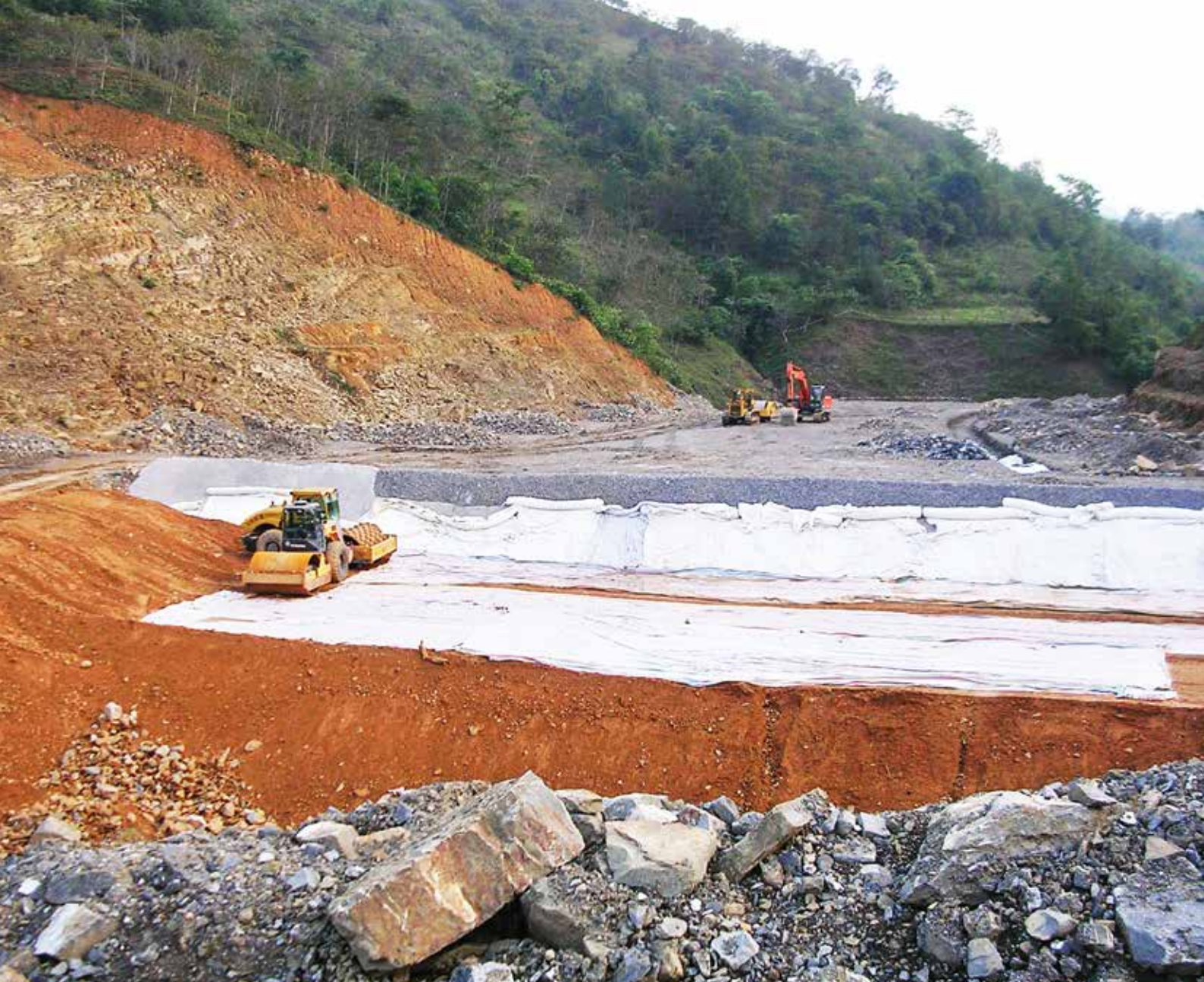
Construction of flotation tailings storage embankment at Jinfeng, China
