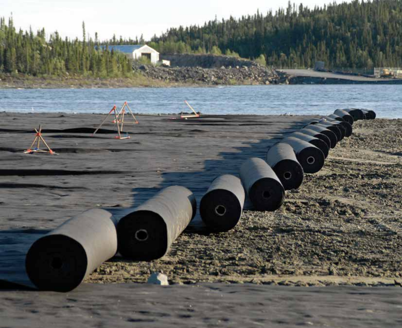
Cover construction over tailings, Colomac Mine, Northwest Territories
