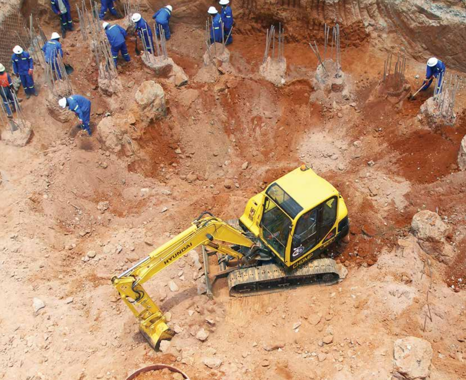
The beginning – surface layout of lateral support and load bearing piles, Konkola, Zambia
