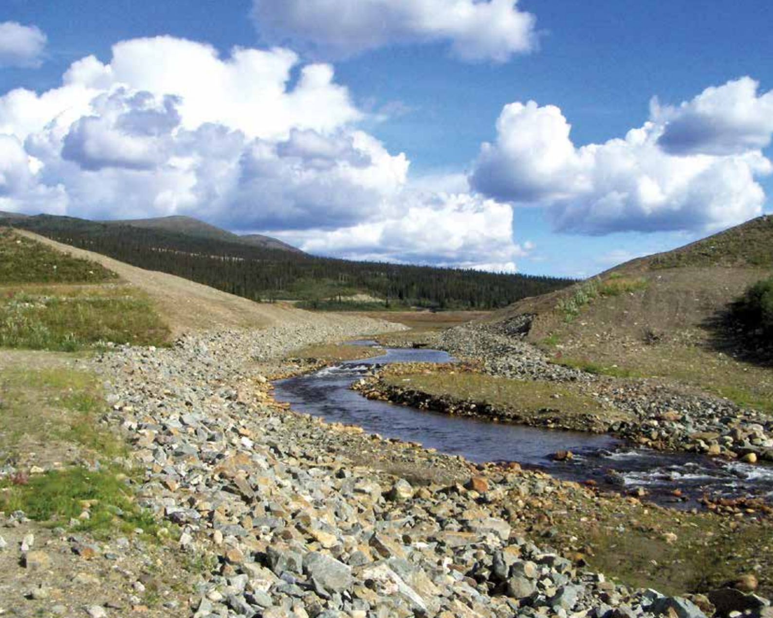
Freshwater supply dam decommissioned to mitigate failure risks, Faro Mine, Yukon. The project included engineered features (i.e. meanders, pools, riffles) specifically designed to create fish habitat within and upstream of the dam breach
