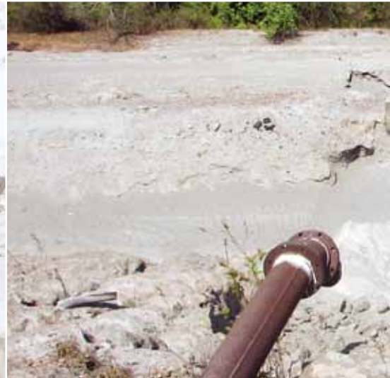
Severe erosion cavity caused by concentrated flow from berm penstock; Broken berm penstock piping causing side wall erosion (right)
