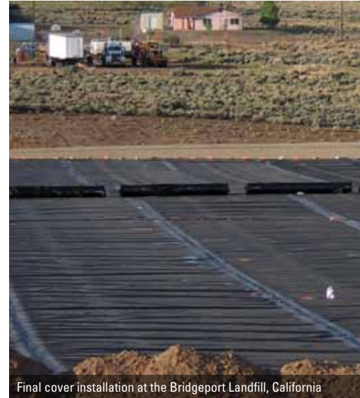
Final cover installation at the Bridgeport Landfill, California
