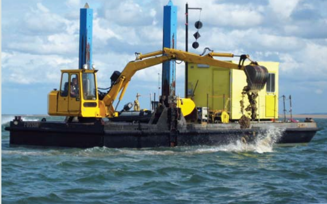
Back hoe dredger at work
