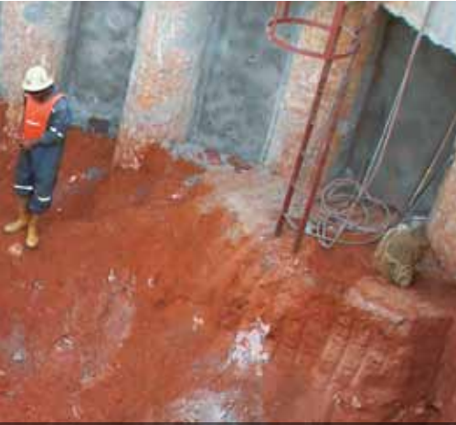
Concrete piles in residual soil to carry the headgear foundation load and provide support during sinking Left: Mini piles in soils above concrete lining
