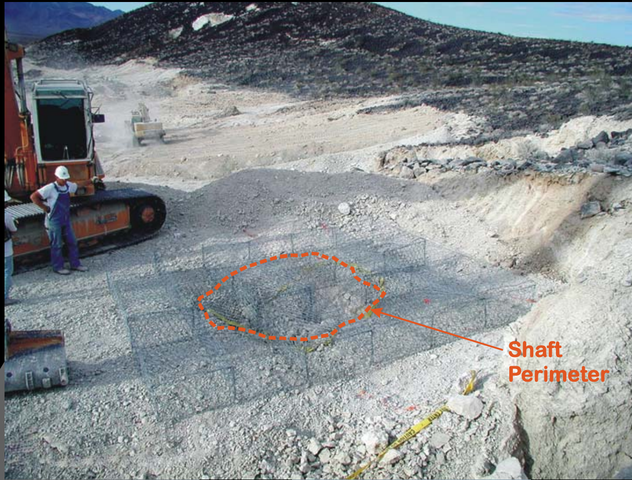
b) First Layer of Gabions of Shaft
