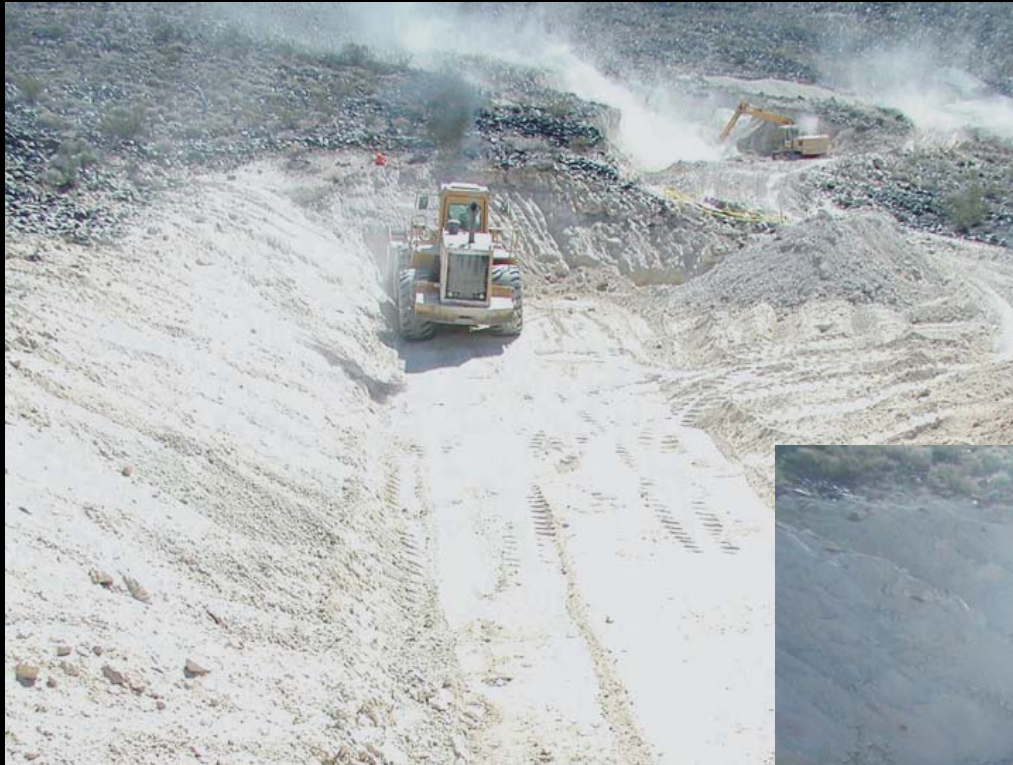
c) Wheel Roll Compaction
