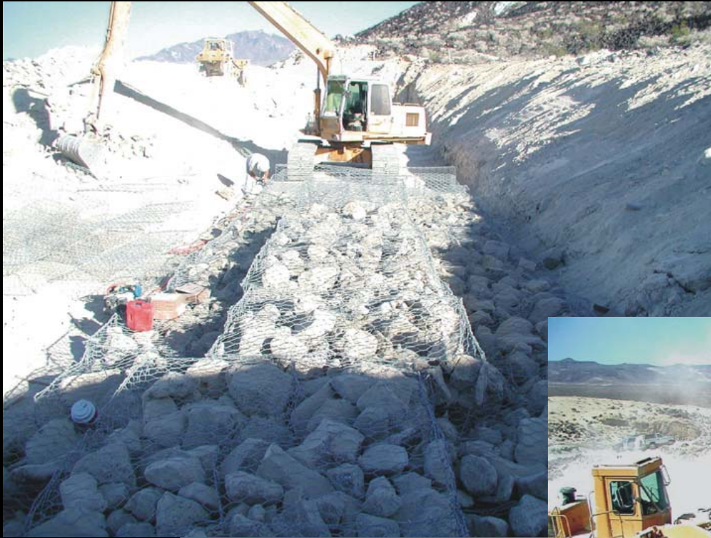
e) Filling Gabions with Native Rock
