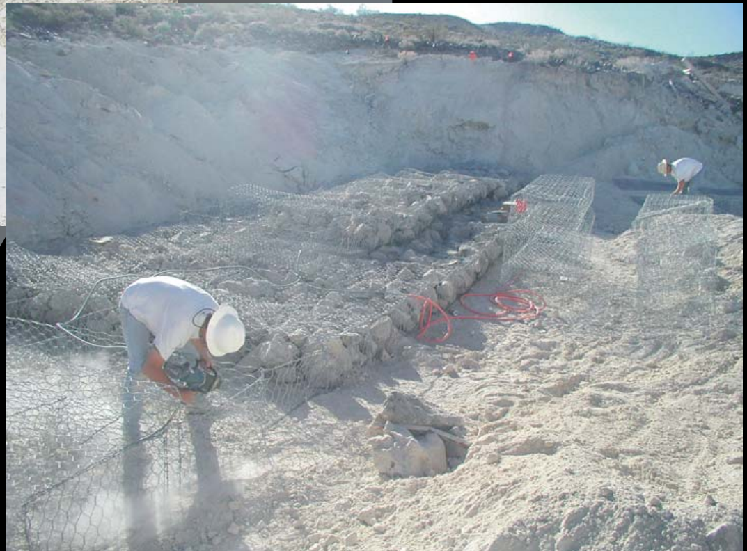
d) Gabion Construction
