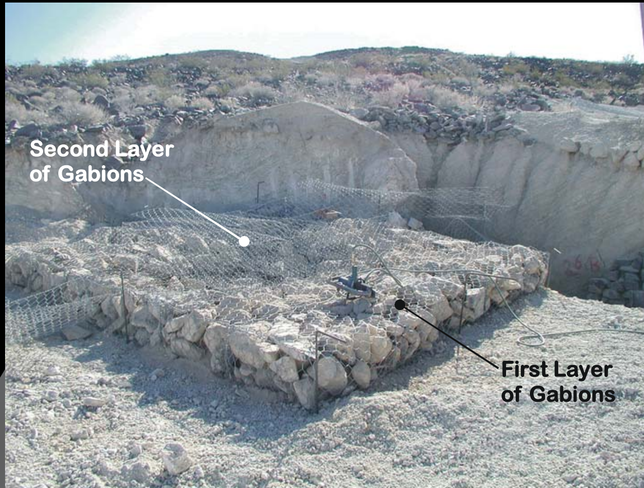
c) First and Second Layers of Rock-filled Gabions— Completed Rock Mattress at Shaft
