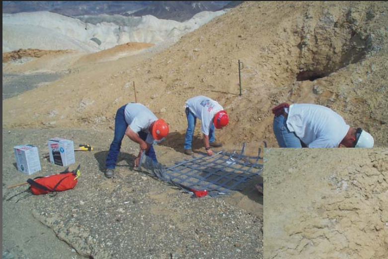
a) Preparing Backing Lattice
