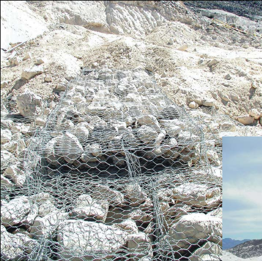
g) Partially Backfilled Rock Mattress
