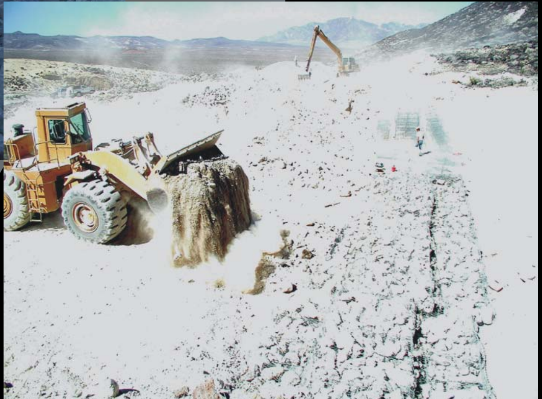
f) Backfilling Over Gabion Rock Mattress
