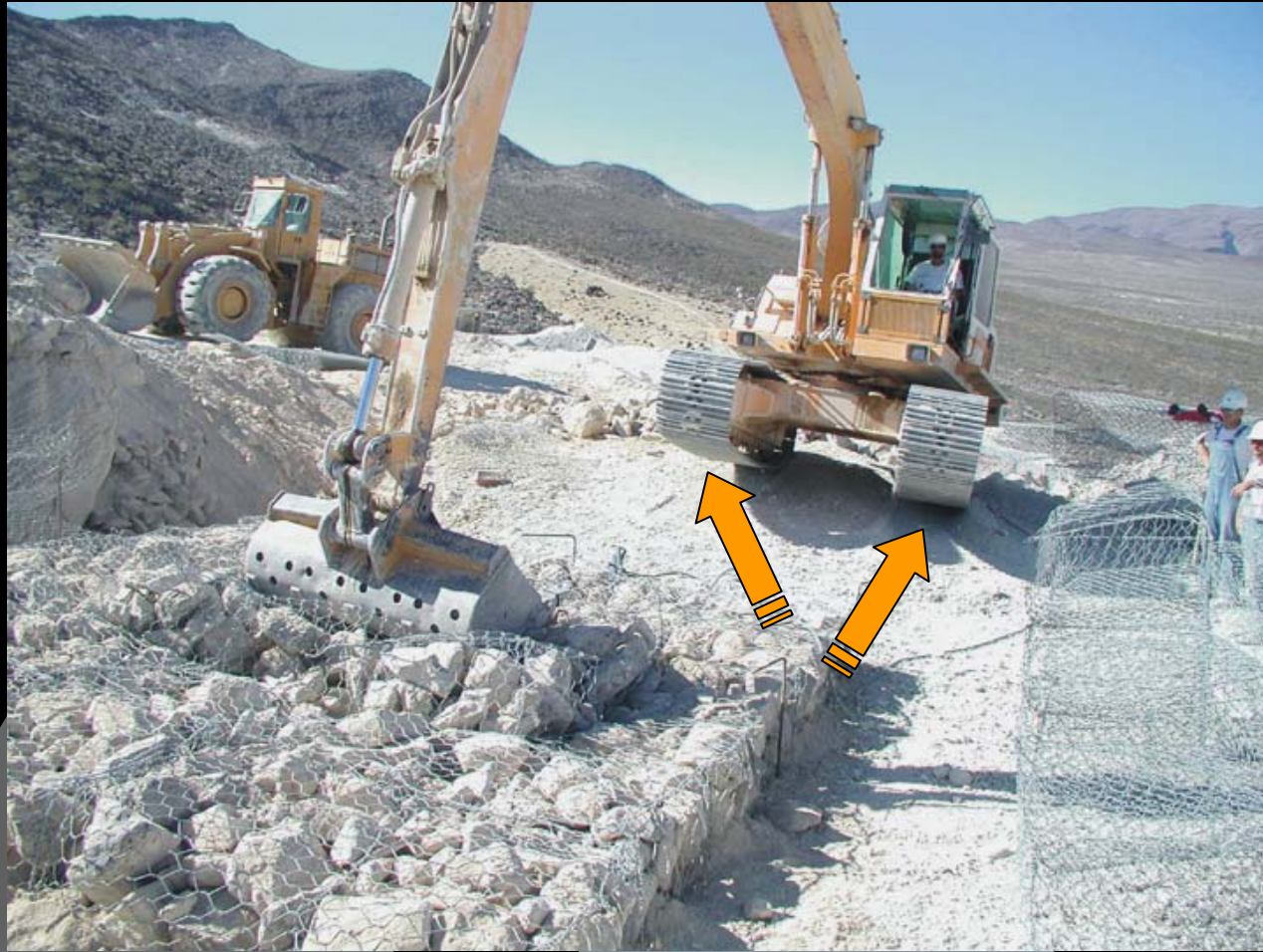
d) “Load Test” on a Rock Mattress at Shaft
