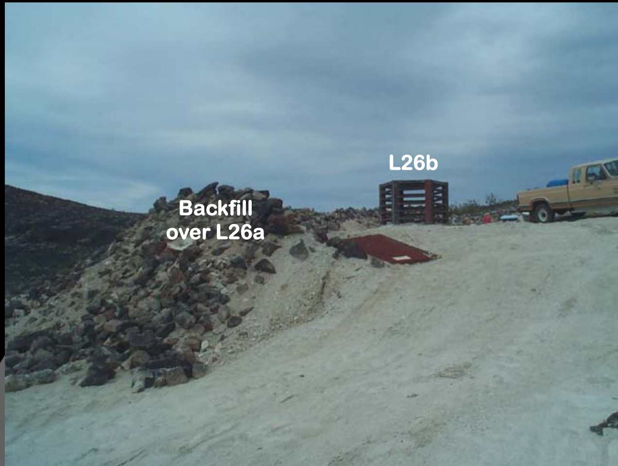
e) Backfill over Rock Mattress
