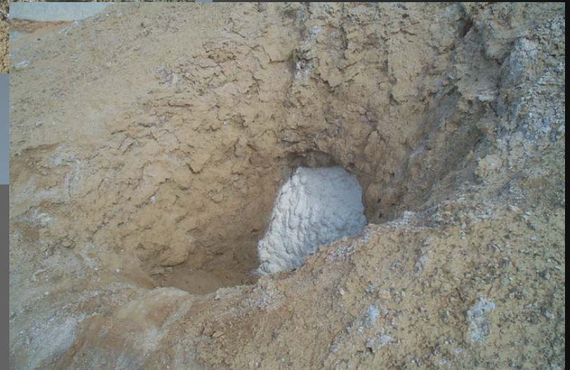
c) Completed Foam Application without Backfill
