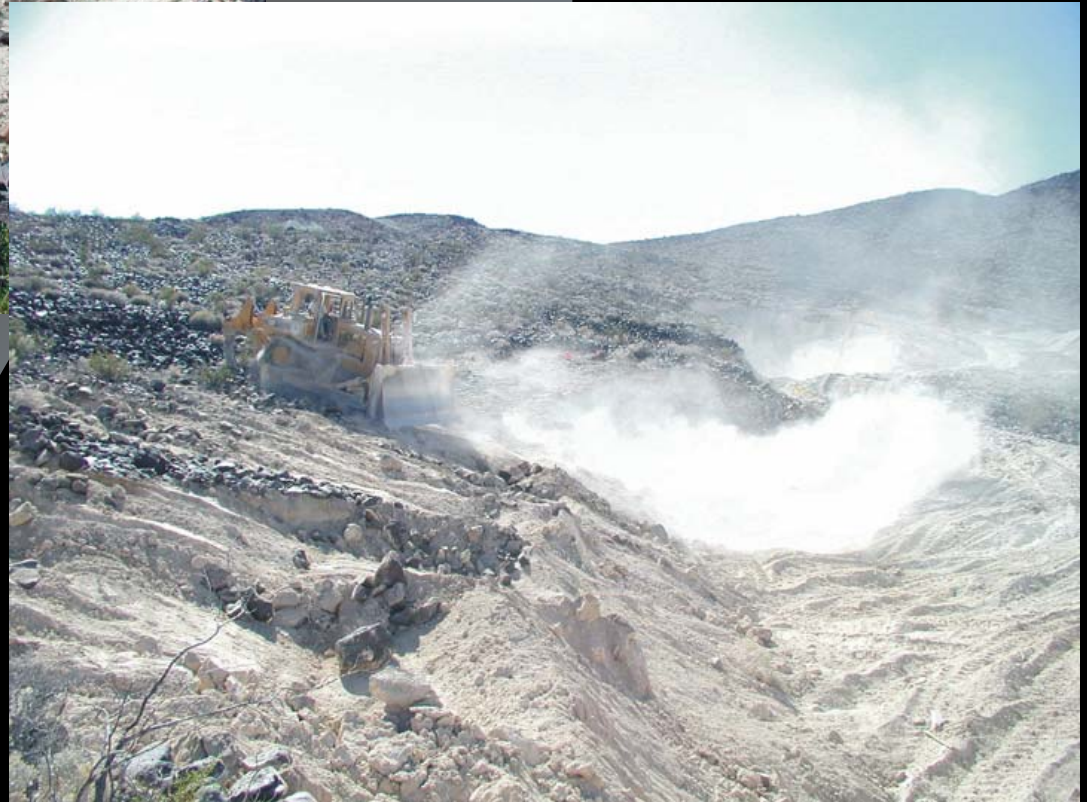
b) Grading Hanging Wall
