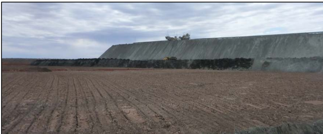
Figure 10: Photograph of successfully implemented preload and buttress, and ripping
