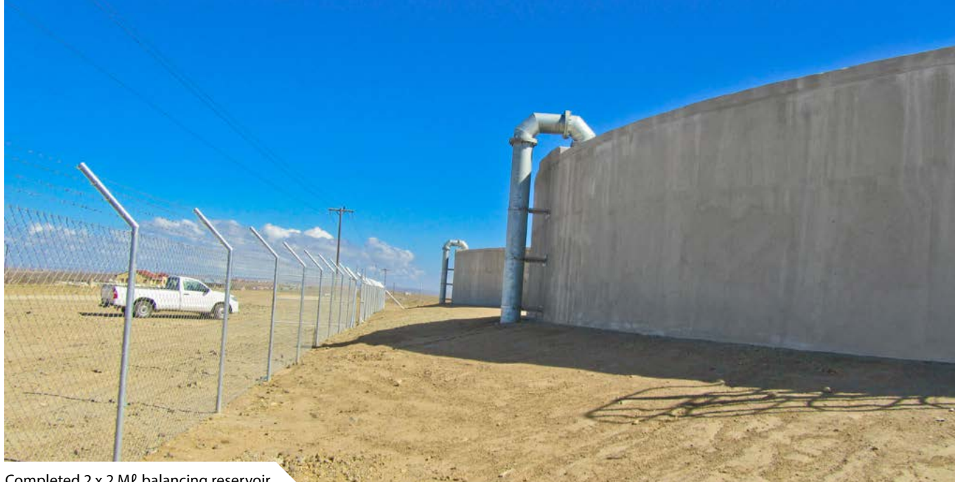
Completed 2 x 2 Mℓ balancing reservoir
