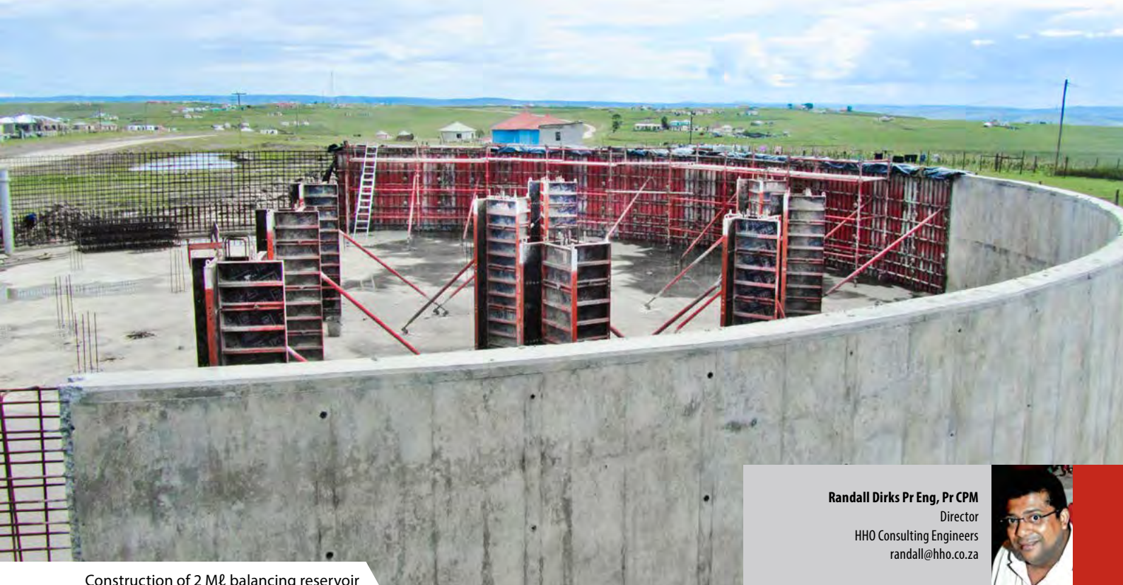
Construction of 2 Mℓ balancing reservoir
