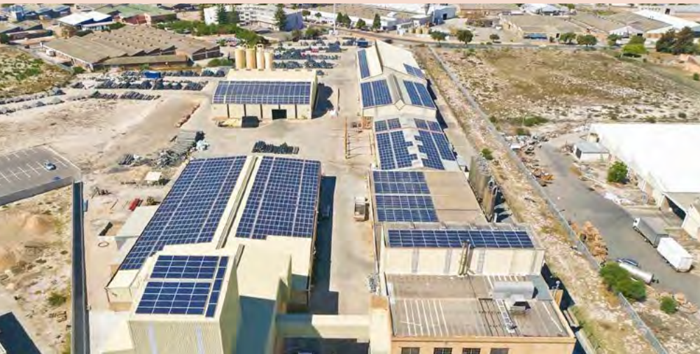
Kaytech has installed 1 947 (315 W) photovoltaic (PV) panels on all the roofs of its Atlantis production facility to optimise sunlight hours, generating about 614 KW during peak exposure time
