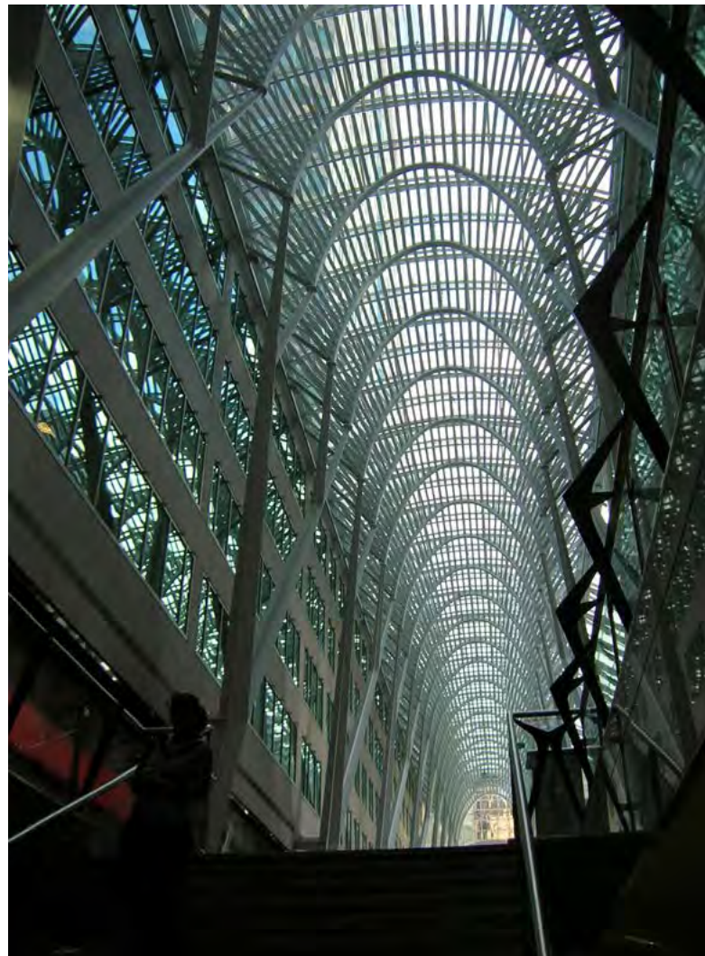
The Lambert Gallery in Toronto (designed by Santiago Calatrava) is an example of a repurposed open area converted to an interior gallery by joining multiple existing buildings, which could complicate evacuation when a fire breaks out
