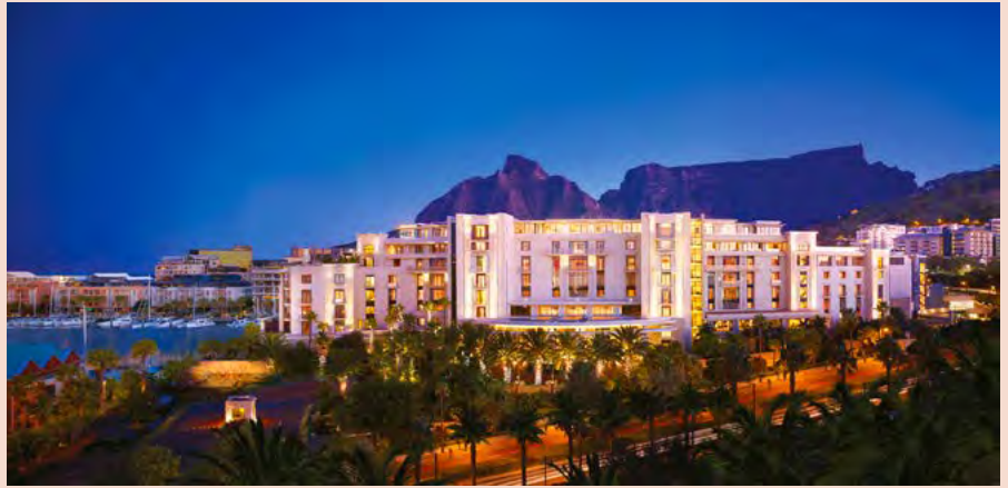
The prestigious One&Only Resort in Cape Town has embarked on an above-ground wastewater treatment facility in a bid to save water
