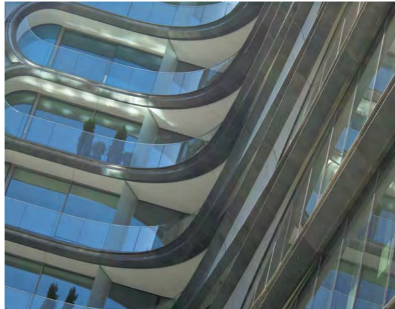
520 W 28th Street, New York – this condominium by Zaha Hadid uses a unique combination of geometry and materials that challenge the conventional control of external fire spread
