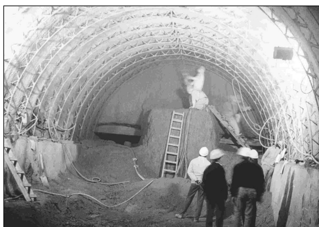
Figure 2. German method of tunneling and first use of shotcrete, Line B, 1998.
