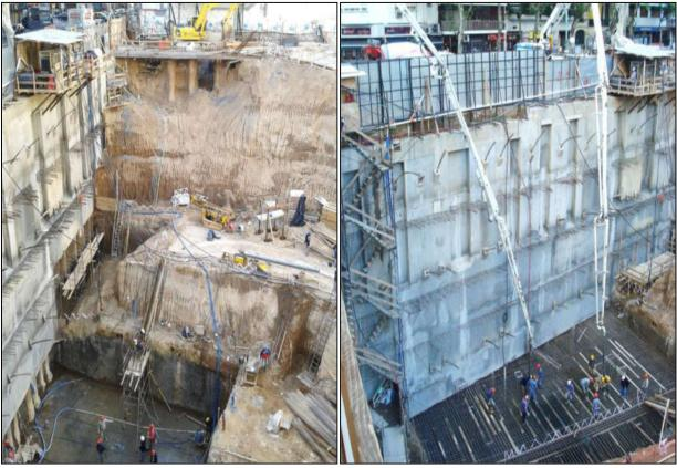
Figure 10. Pile-supported excavation, street side of Vista Tower.
