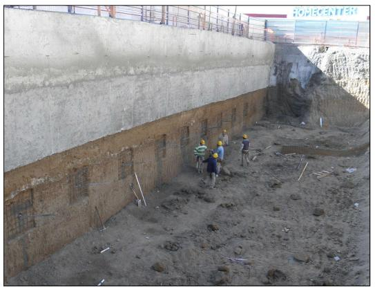
Figure 15. Detail of one excavation stage. Note the carving and mesh reinforcement for the anchor plates, and the ground surface waiting for the shotcrete to be placed.
