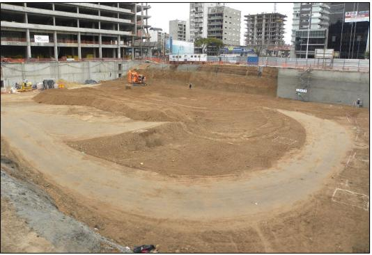
Figure 14. Overall view of the excavation of the Al Río project in Rosario, Argentina. Note the wall supported with shotcrete and ground anchors, and the buttressed portion to be excavated.
