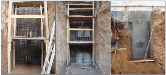
Figure 7. Construction sequence of the anchor plates as part of the final wall (Laría 2015).
