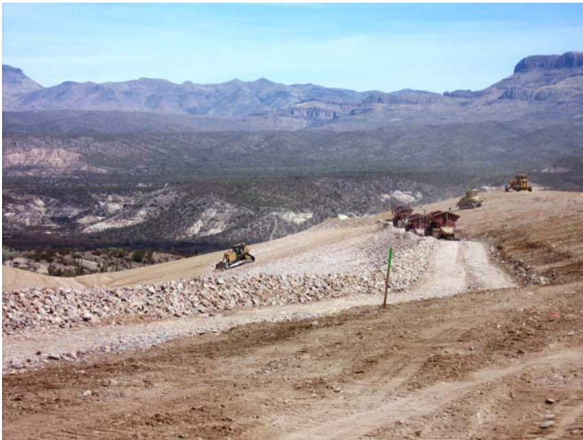
Photo 4: Installation of rock armor on 6 Dam
