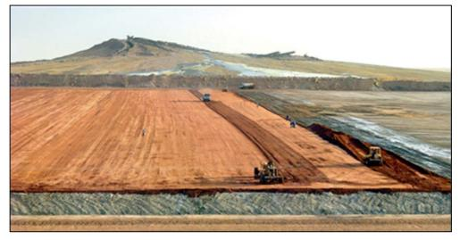
Placement of the clay liner during leach pad construction in Niger
