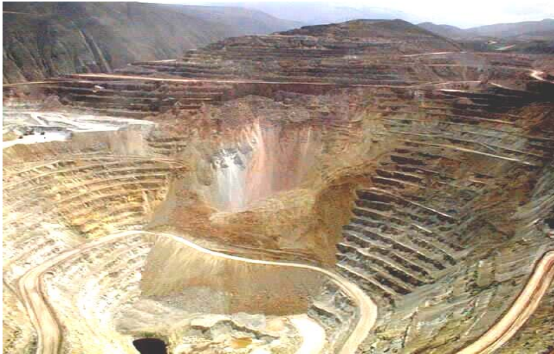
Figure 4 East wall failure (D15) at Cuajone Mine in 1999
