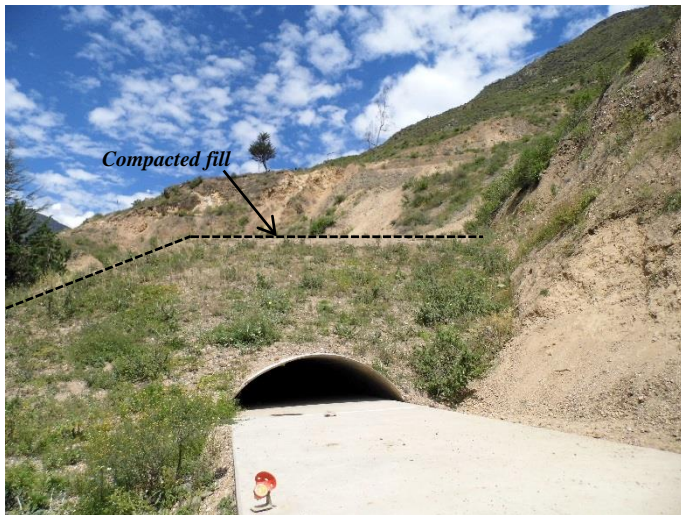
Figure 16. Filling at the toe of the landslide – April 2016.
