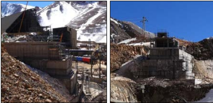
Figure 2-7. Concrete buttress for foundation restitution at the main power plant.
