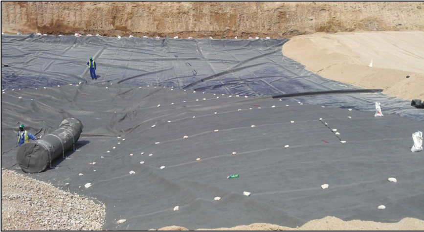
FIG 8 – Collection sump during construction.
