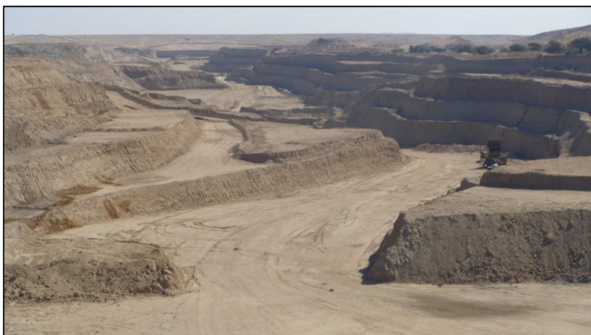
FIG 4 – Photograph of mined out pit with partial palaeochannel reinstatement.
