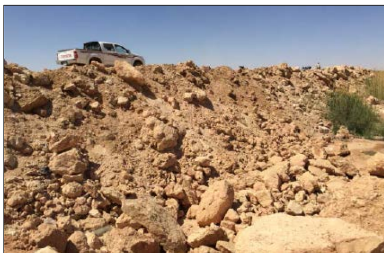
Figure 5: Typical grading of overburden material used for embankment construction
