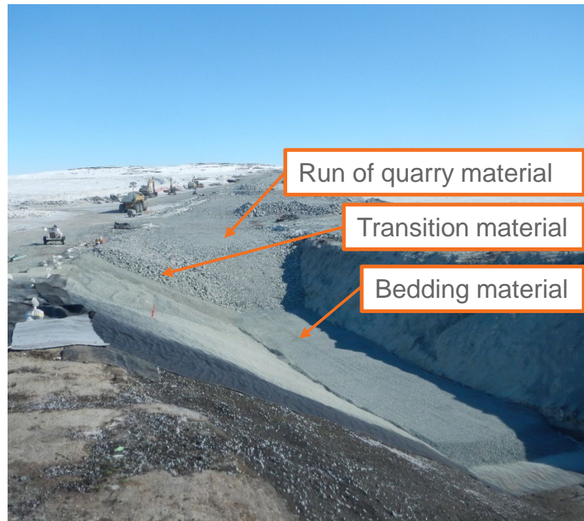
Backfilling of key trench above liner
