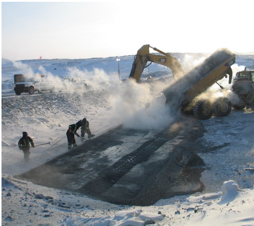
Frozen core construction
