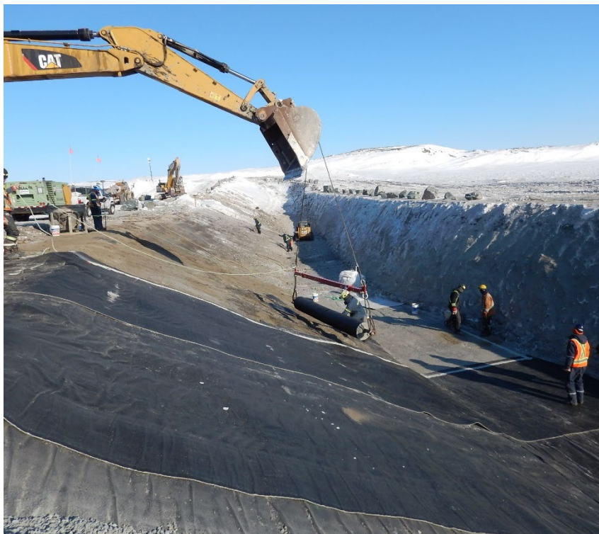
Deployment of liner on upstream slope of key trench
