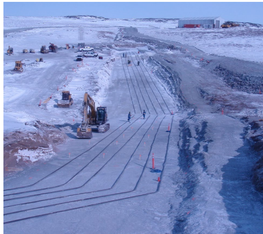
Thermosyphon evaporator pipes installed along the key trench base
