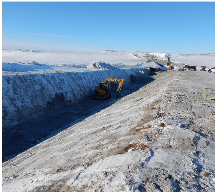
Near complete section of key trench
