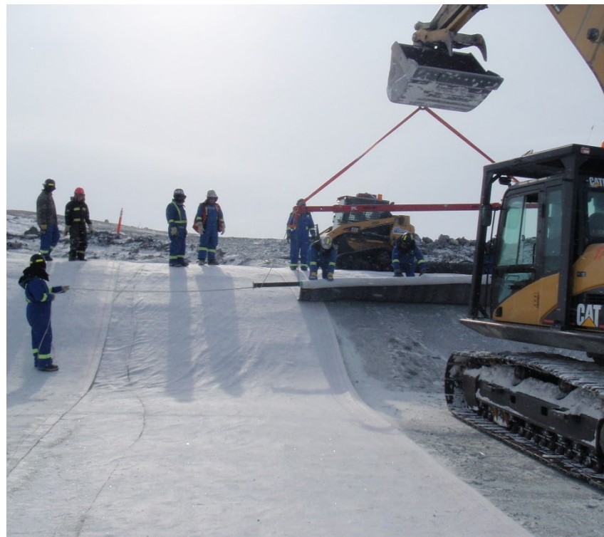
Liner installation in key trench
