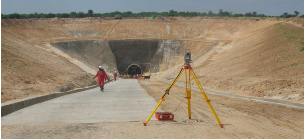
Figure 4: Panorama of the completed box cut showing graded slopes, December 2011.
