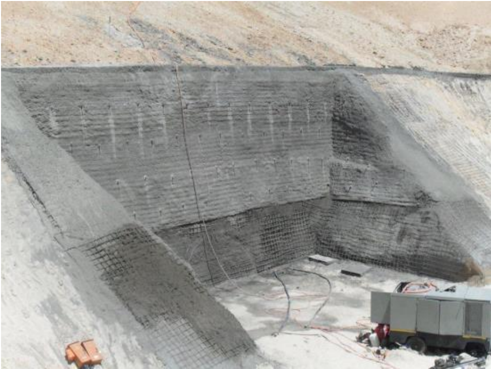
Figure 6: Portal construction showing mesh installation prior to shotcrete placement.
