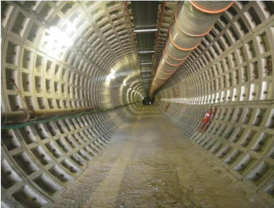
Figure 11: General view of the segmental concrete lining in the decline shaft.
