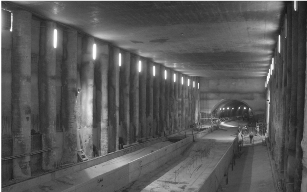
Figure 10. A cut&cover cavern completed..
