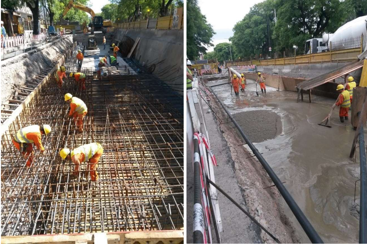
Figure 36. Pre-Hospitales tunnel. Construction of roof slab and filling with CLSM.
