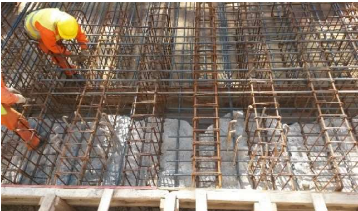
Figure 35. Pre-Hospitales tunnel. Connection of the slab reinforcement to the piles.
