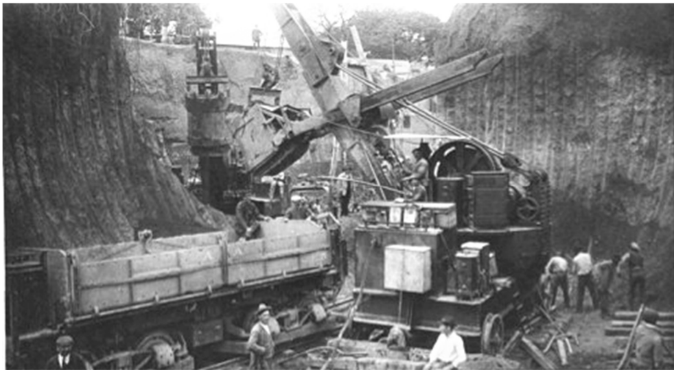
Figure 1. Excavation of Line A in 1911 (SBASE 2017).
