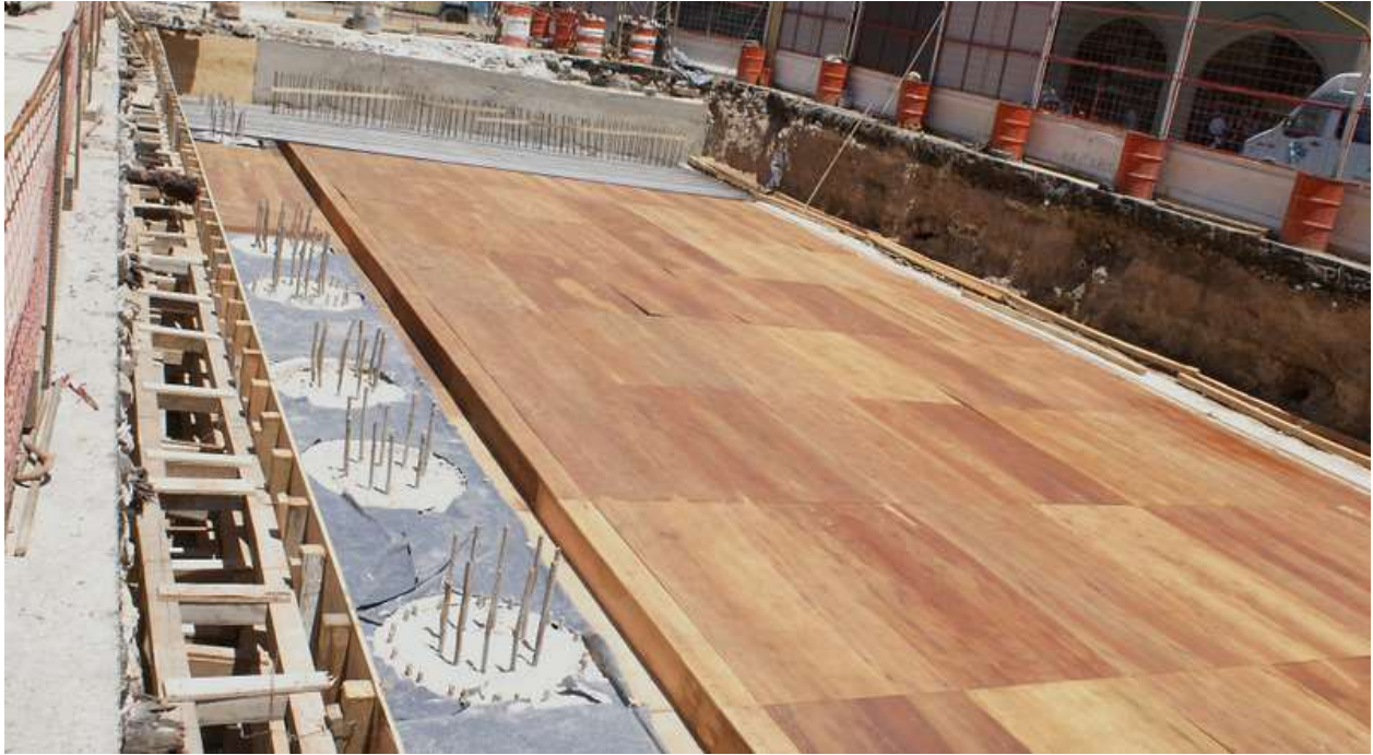
Figure 23. Correo Central Station. Construction procedure of the roof slab-on-piles.
