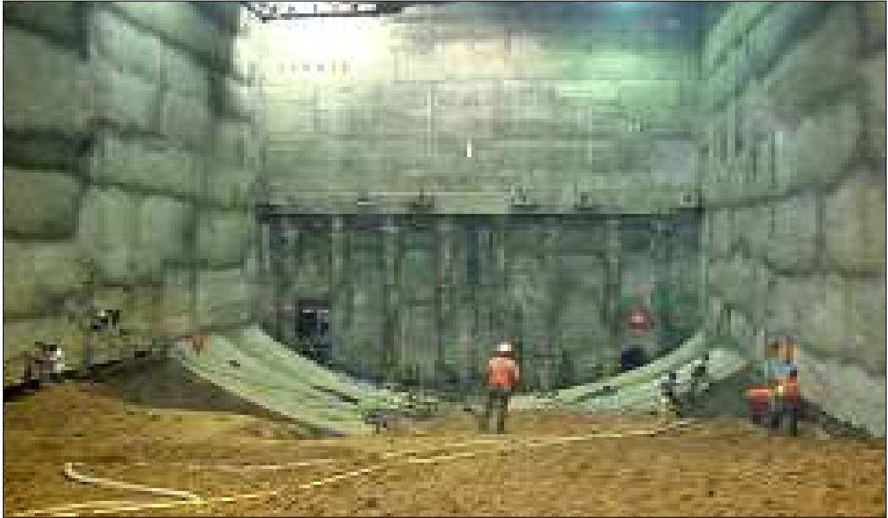
Figure 25. Correo Central Station. Phase 2 excavation, pile-supported wall and invert.
