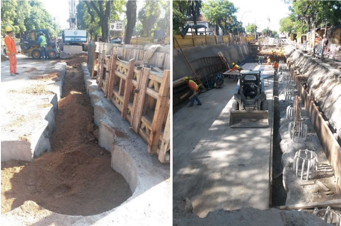
Figure 34. Pre-Hospitales secant wall. Construction of concrete template and finished wall.
