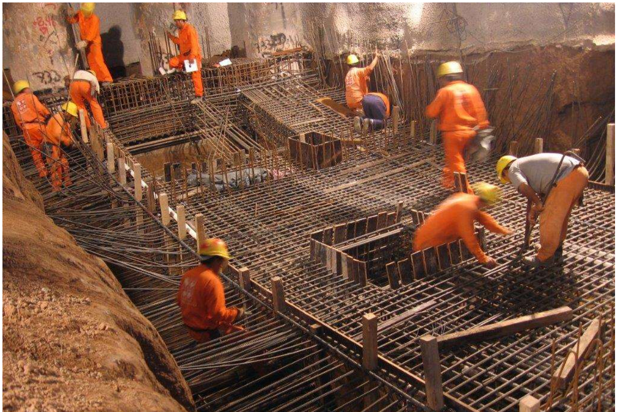
Figure 29. Strip excavation of the invert.
