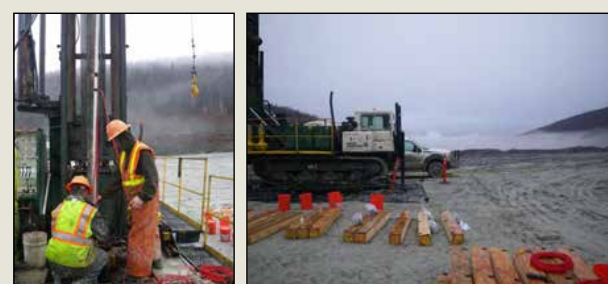
Sonic drill rig used for recovery of core and installation of VWP at boreholes SB-1, GP-1, and RR-1
