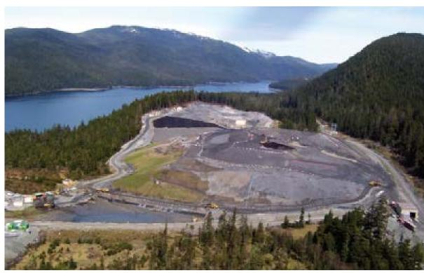
**Operator:** Hecla Greens **Creek Mining** Company **Operating:** 1989 - present Mill throughput: 2,200 tons/day **Total capacity:** 13 million tons
