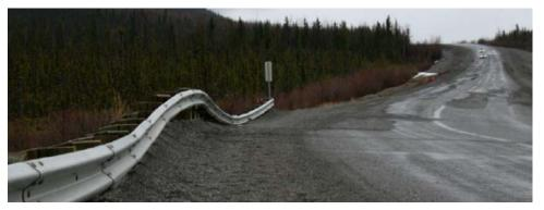
Differential thaw-settlement of a highway caused by degrading permafrost.
