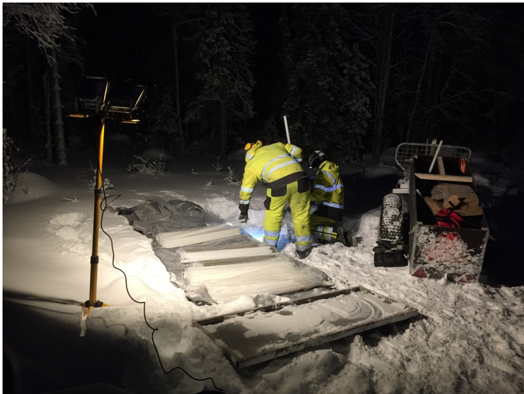
Figure 3: Preparing for a Smartwell installation
